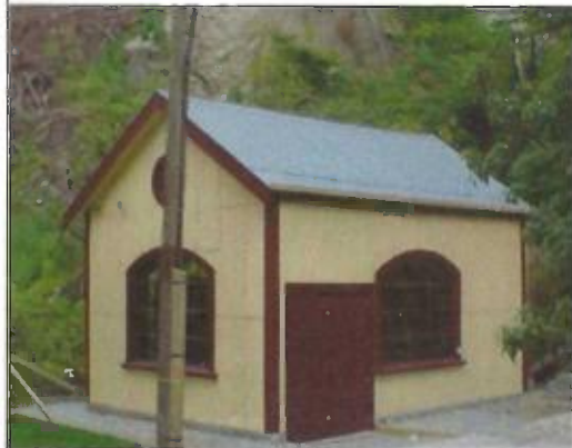
The Power House was saved from ruin and reopened in 2005 as a static museum display after restoration work administered by the One Mile Restoration Trust. Photo: Malcolm Boote
